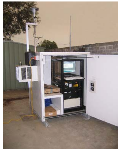
Figure 3: Mobile air monitoring station at Bairnsdale, 9 December 2006
