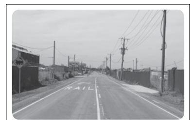
Bunting Road in Brooklyn. Before and after recent road sealing works.
