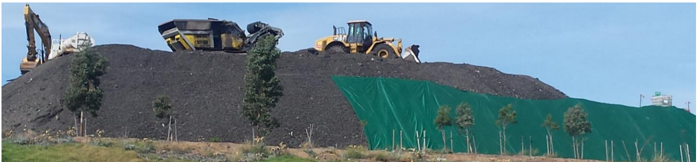
Figure 7: Stockpiles being covered under tarpaulins Source: Fulton Hogan
