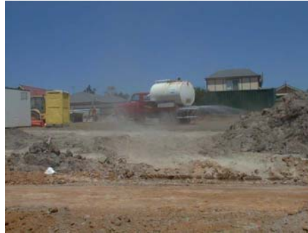
Photo 5: Dust Suppression by Watercart
