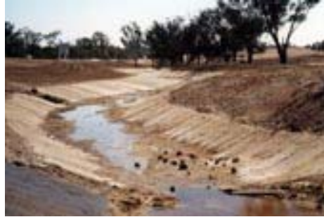
Photo 9: Stabilisation Matting Used to Stabilise Drainage Channel (Courtesy of Treemax)
