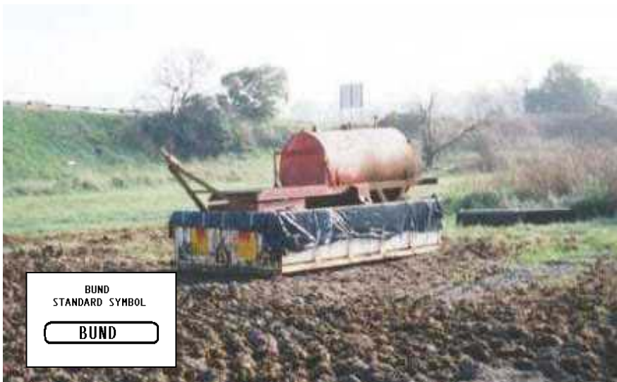
Photo 40: Lined Trailer Utilised as a Bund
