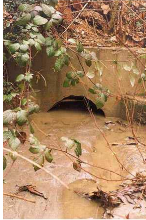
Photo 6: Sediment Deposition
