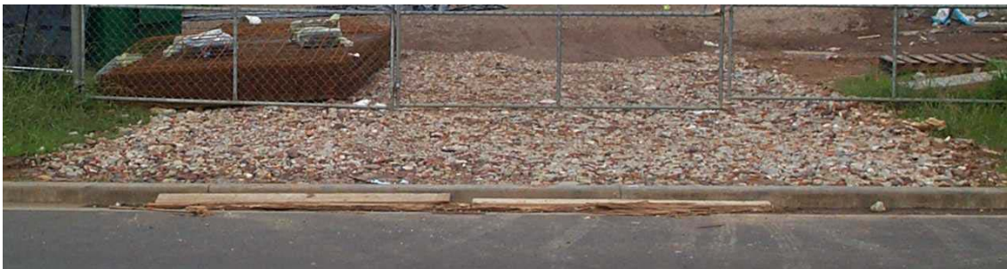
Photo 34: Stabilised Access Point (courtesy of Tony King, CPESC)
