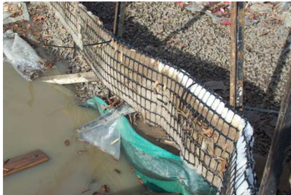
Photo 22: Trapped Sediment Visible on a Composite Silt Curtain (Silt Cell) During Low Flow Conditions
