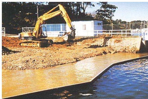
Photo 20: Floating Silt Curtain (Courtesy of Geofabrics Australasia)
