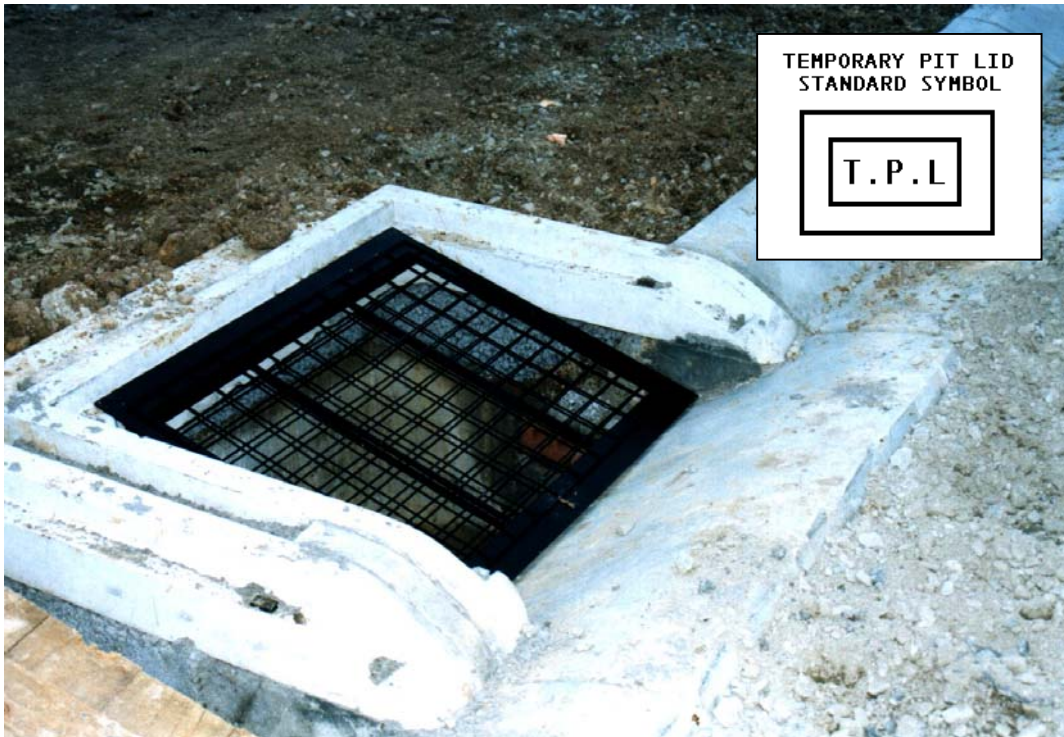
Photo 28: Temporary Pit Lid (without geotextile cover)
