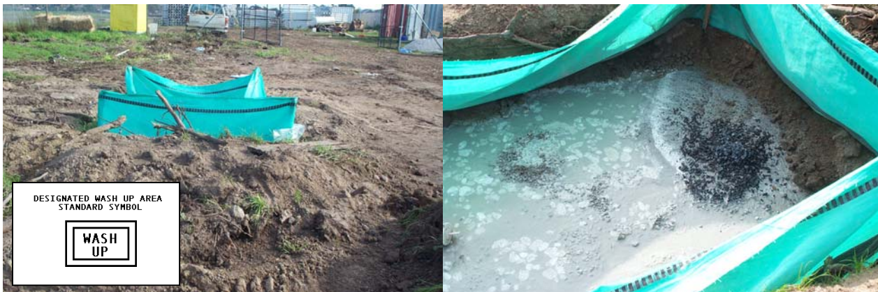
Photo 39: Designated Concrete Washout Area
