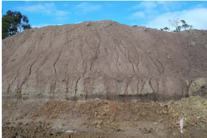
Photo 12: Eroded Stockpile
