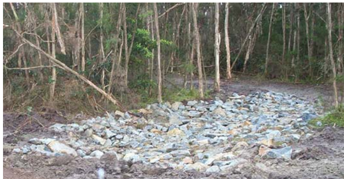
Photo 10: Rock Armoured Drainage Channel
