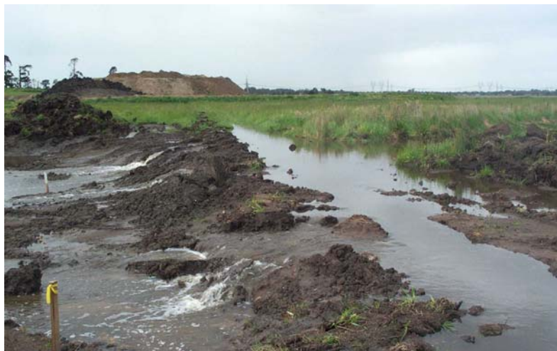
Photo 7: Breach of an Undersized Catch Drain
