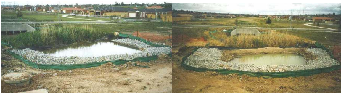
Photo 21: Rock Bund Across Creek (a) During High Flow Water is Able to Overtop (b) During Low Flows Captured Sediment is Visible
