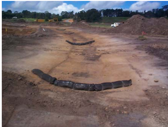
Photo 18: Synthetic Log (courtesy of Statewide River and Stream Management)
