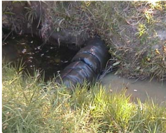
Photo 17: Synthetic Straw Bale Replacement (courtesy of Statewide River and Stream Management)
