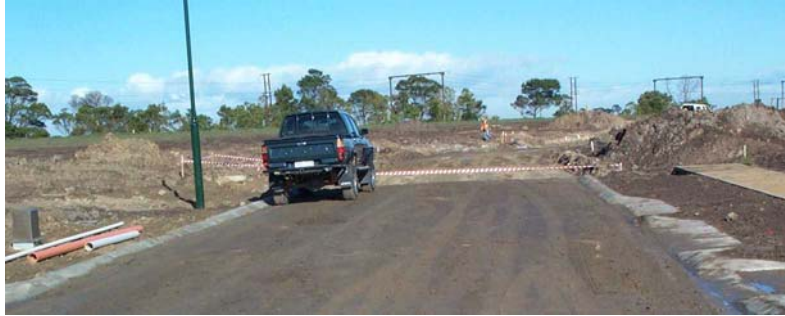
Photo 33: Barricaded Access Point
