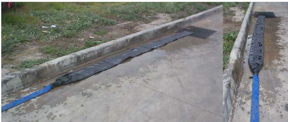
Photo 37: Pump Sack (Courtesy of Statewide Streams and River Management)
