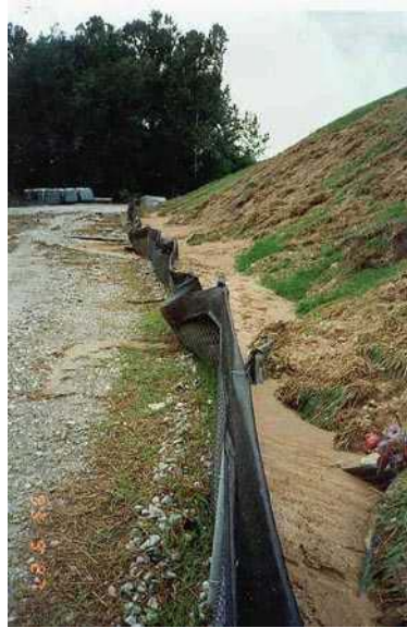
Photo 11: Silt Fence at Base of Stockpile
