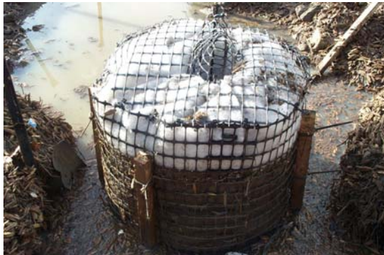
Photo 23: Synthetic Silt Filter Around a Standpipe
