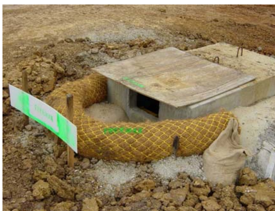
Photo 26: Coir Log Utilised for Inlet Protection
