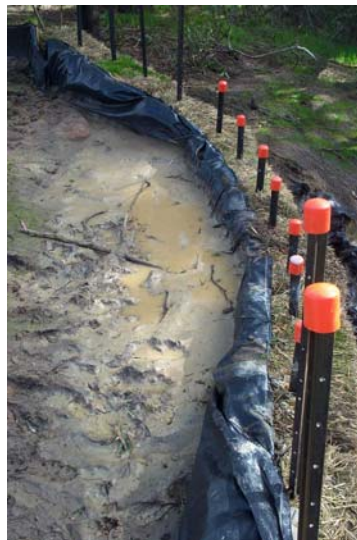
Photo 15: Sediment Retained by Silt Fence and Straw Bale Sediment Fence
